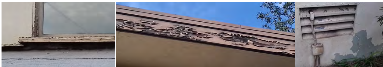
Peeling paint, eroded window fittings, cracks in stucco, and evidence of dry rot are all indications of repairs that are long overdue.
